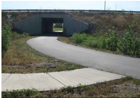
Pedestrian/Bike Tunnel under MacArthur Blvd.
