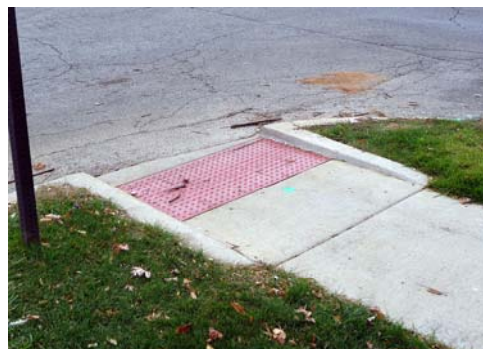
Fully accessible detectable ramp
